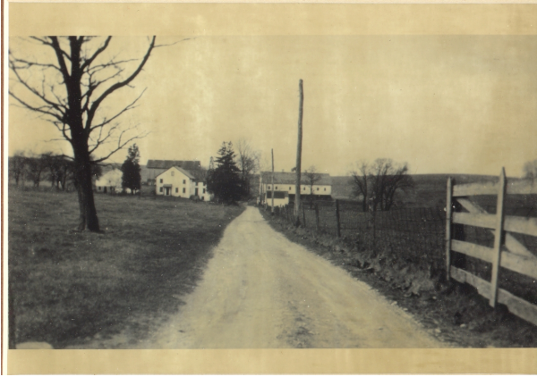
Figure 07.1: Looking down the lane to the farm on Second Lock Road
