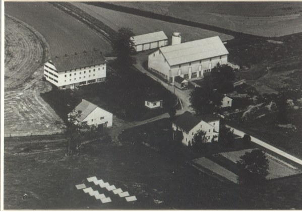
Figure 07.6: Aerial view of the Hess farm on Second Lock Road
